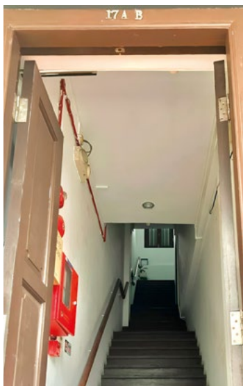
17A Keong Saik Road looks different today from its 1970s notoriety without the red and white light box. Photo taken by the author.
