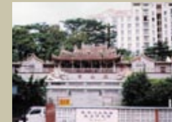
8. HONG SAN SEE TEMPLE LOCATION 31 Mohamed Sultan Road (Gazetted on 10 November 1978)
