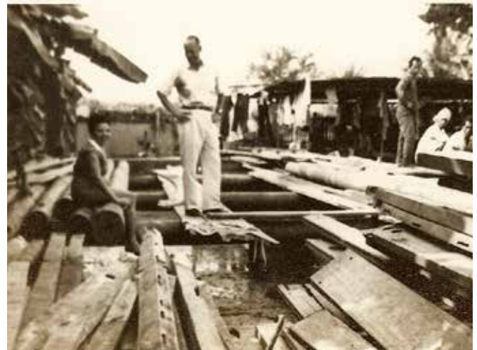
Connie and Jim when the house was under construction
