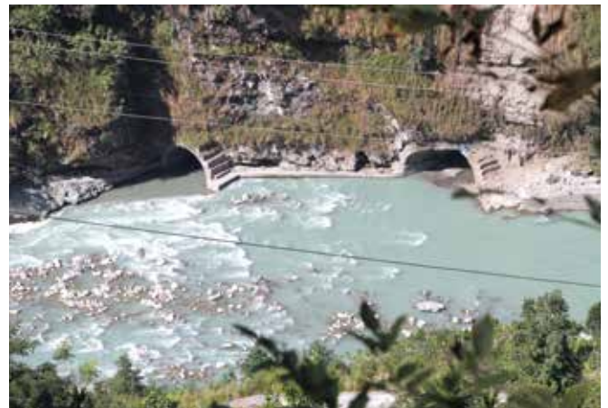
Diversion tunnels through the mountain
