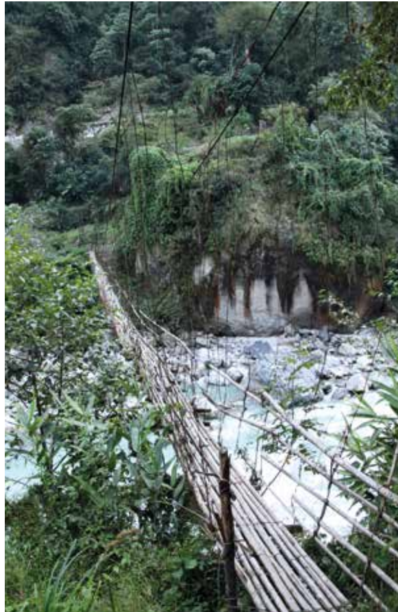
A bamboo suspension bridge in Dzongu
