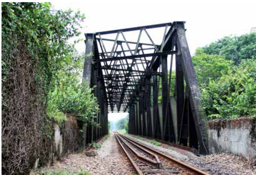
The Truss Bridge close to Bukit Timah Railway Station
