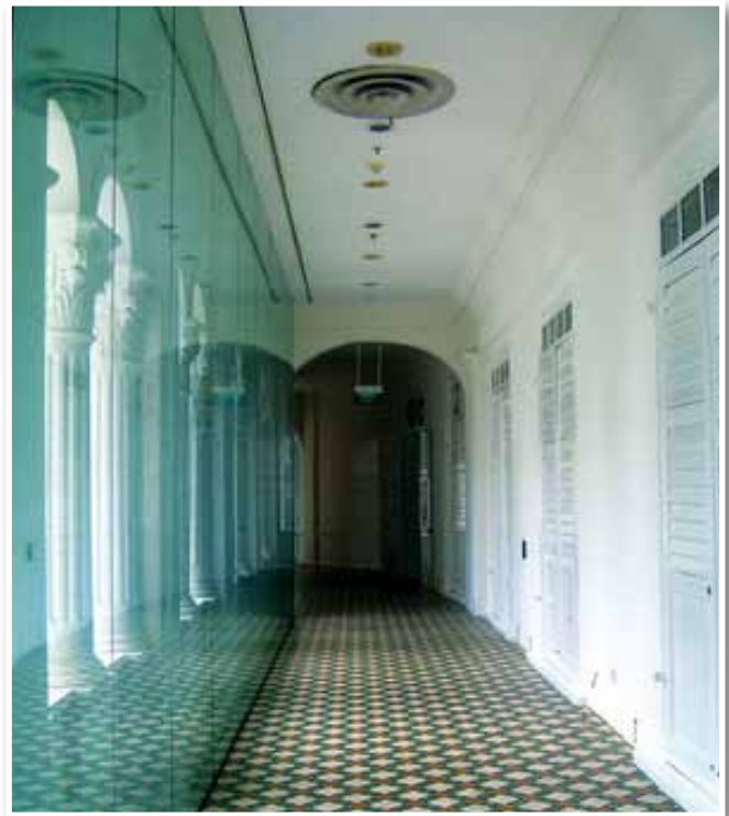
Corridors with shutters and glass inner shell
