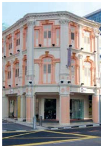
Restored China Square shophouse with a local interpretation of the Palladian window and columns, which run the full length of the façade
