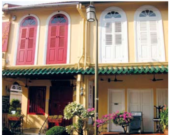
Transitional Style shophouse in Club Street with Georgian fanlights above the louvre windows
